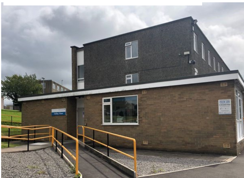
Figure 2 - Valley View at West Cumberland Hospital
